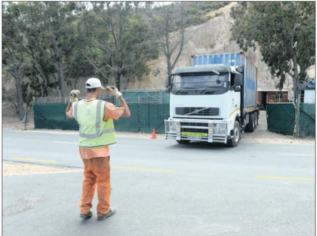
NEW MOVE: A container is removed from the site on Chapman's Peak where the toll company, Entilini, plans to build its headquarters. Picture: MICHAEL WALKER
